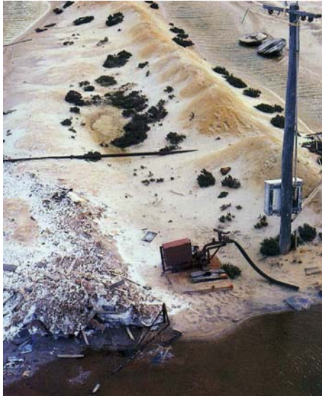
Figure 8.5 - Bourka 8005 site. The bore with pump attached is in the foreground.
