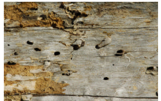
Picture: EHB emergence holes (running with the grain of the wood) and blisters caused by frass
