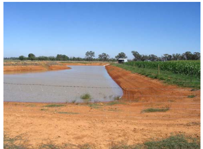
Figure 2 Storage, pump shed and suction – note the fenced-off storage
