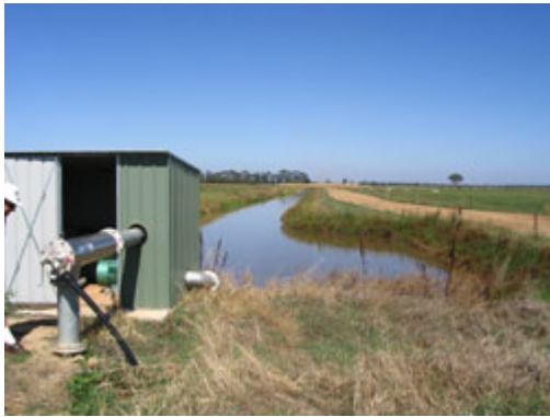
Figure 2: Water storage, filter and motor to operate a centre pivot system
