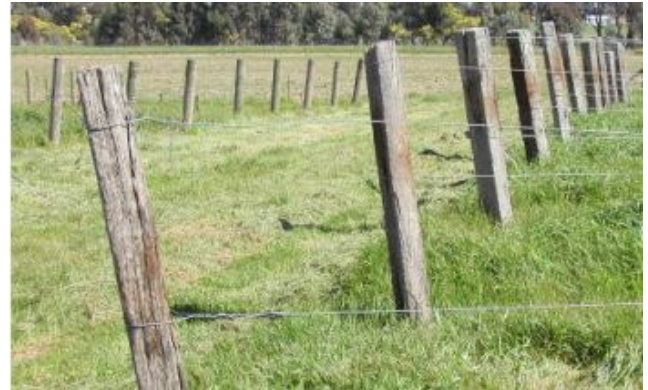
Untreated heartwood timber from durable hardwood species makes suitable vineyard trellis posts.
