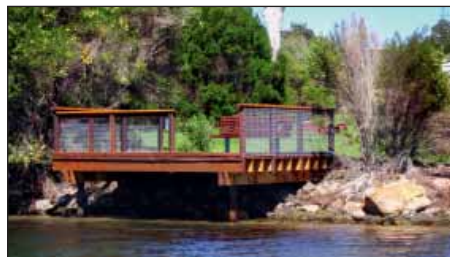
Project complete: $75,000 towards three fishing platforms at Mallacoota.
